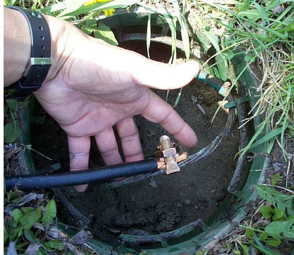
Connection to existing ground electrode
