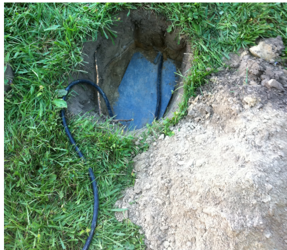
Ground Plate installation
